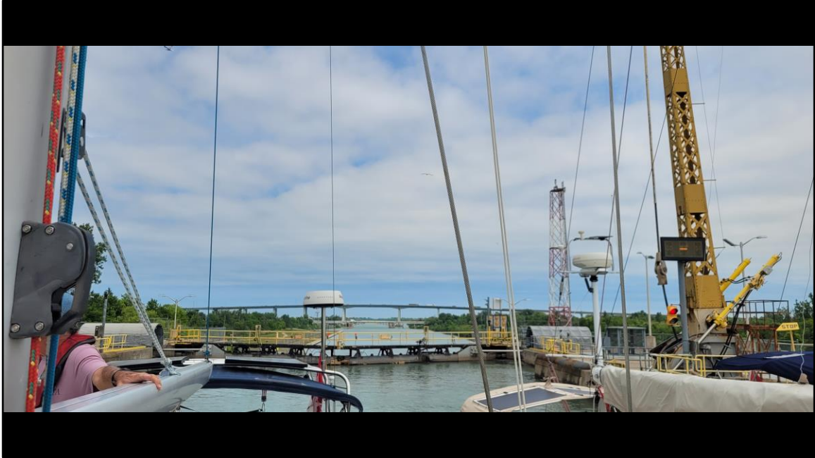
Lock 3 looking back at Queenston Road Bridge and the QEW Garden City Skyway
