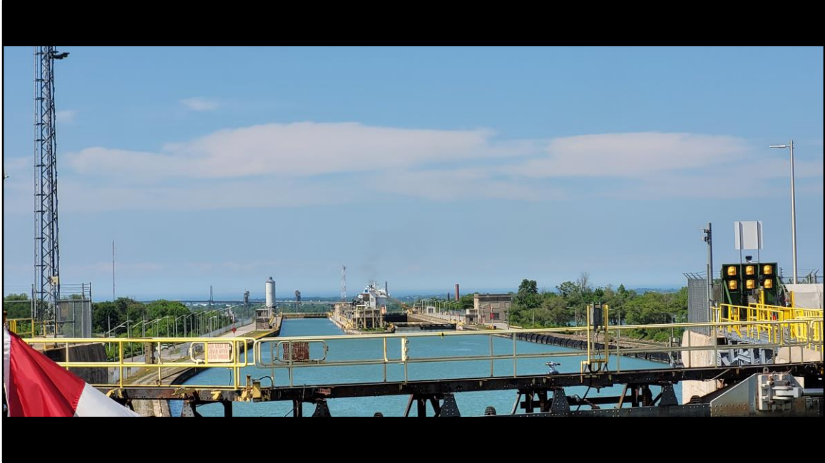
Inside Lock 7 looking back at Lock 6 (the top of the Flight locks and the Niagara Escarpment)
