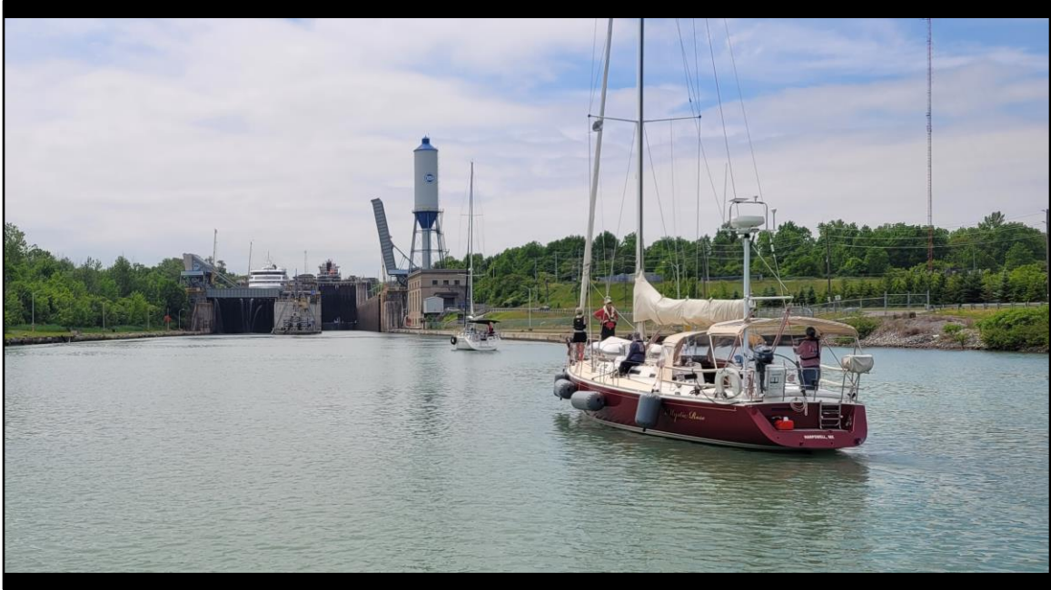
Mystic Rose approaches Lock 4 – Graham & Diane on the bow. The "water tower" at Lock 4 is actually a differential surge tank for the Lock 4 Powerhouse, a hydroelectric generating station that provides power for the canal's operations.
