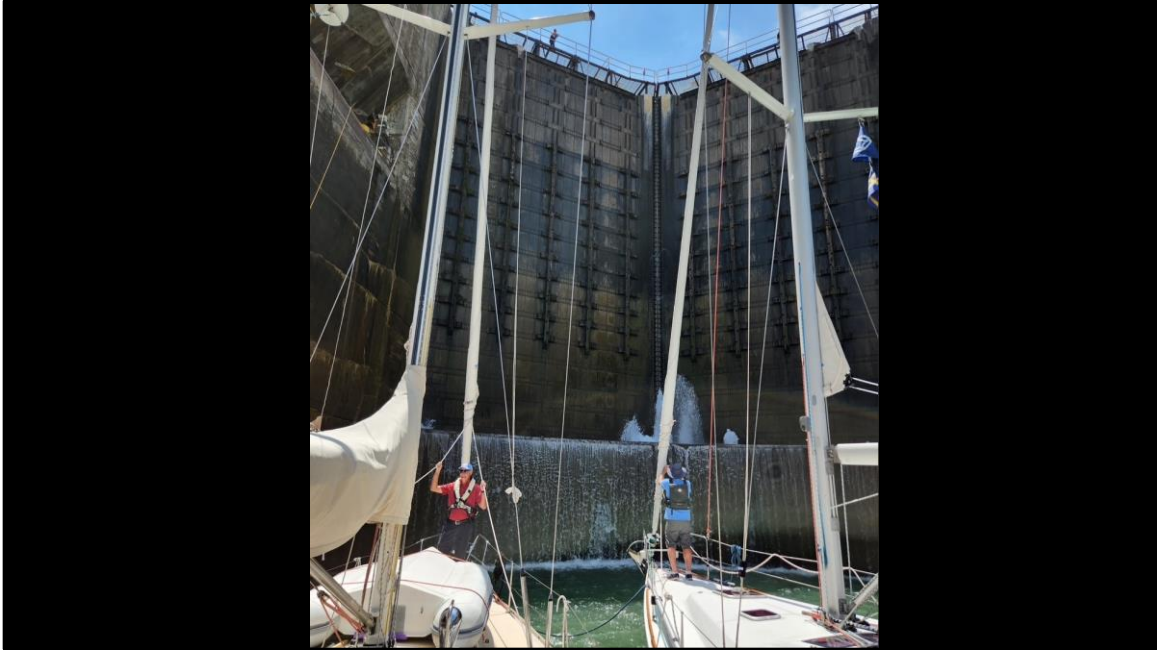
Graham and Bill in the Flight Locks (4, 5 & 6). Lock doors are double height because the locks are back-to-back. These three locks are also twinned meaning there are parallel locks and boats can pass going up and down the canal.
