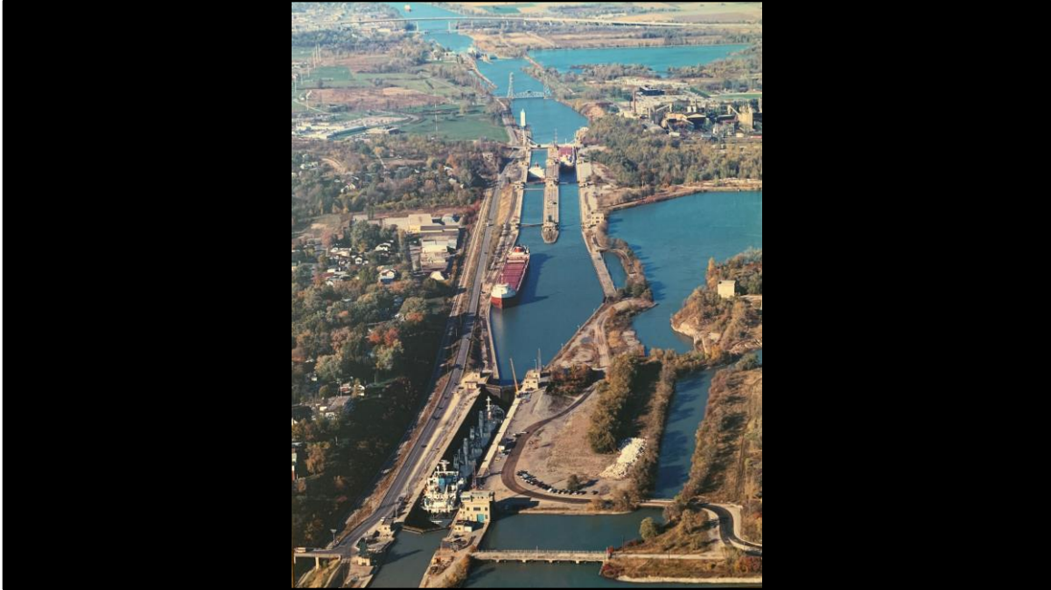
Looking north; Lock 7 in foreground, 3 flight locks; Glendale Bridge; Lock 3; Skyway Bridge
